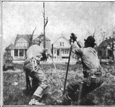
Fig. 11.—View Showing Method of Straightening Pole.
